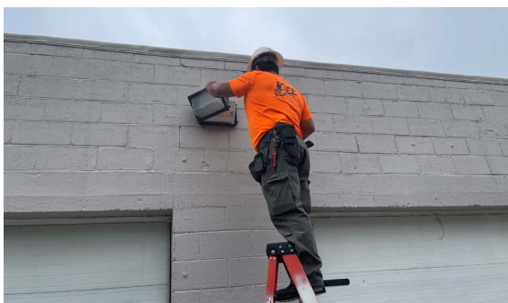
Gus Bautista (Bee Electric) updating exterior lighting
